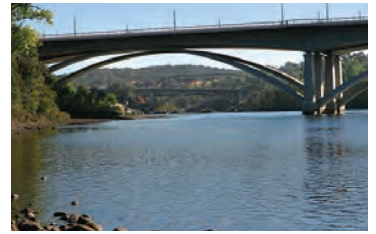
New Folsom Lake Crossing Bridge
