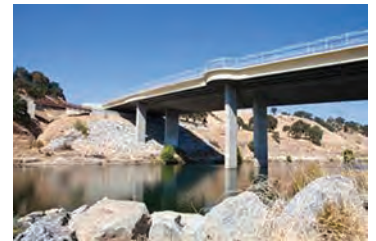
Hazel Ave expansion and bridge improvement in Fair Oaks
