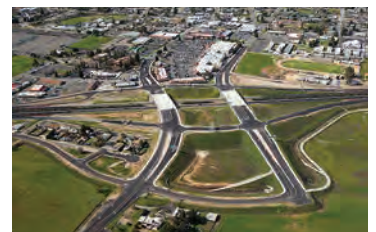
Hwy 99/Central Galt Interchange improvement
